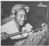
BOLTS ARE tightened through the use of a foot-pound torque wrench. BOLTS TA worde cerrá usando un yabi di torque cu ta marca foot pounds.
